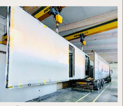
More and more prefab companies are offering panelised systems that are easy to transport and assemble, and make for a fully insulated building envelope that significantly reduces heating and cooling needs. Image: Zen Haus Group
