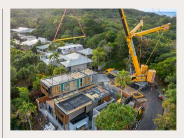
With a prefabricated approach, most of the construction work is done before transportation, minimising time spent onsite. Here, a module by Prebuilt is craned into position in Byron Bay, New South Wales. Image: Media Drive
